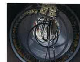
SPR-SE 工法 SPR-SE Method
